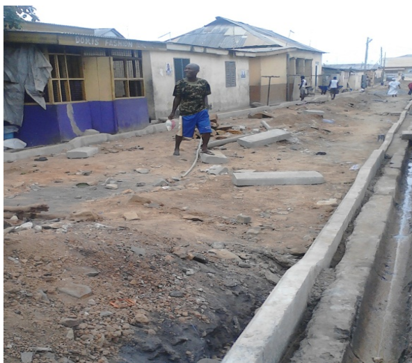
Figure 9: drainage Canals along the Alleys to Mitigate the Effects of Flooding in Ga Mashie
